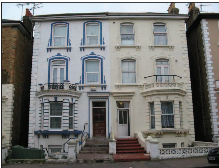
These properties in Athelstan Road would benefit from grant aid to restore lost architectural features
