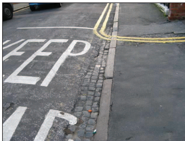
Granite setts and kerb detail, Ethelbert Road
