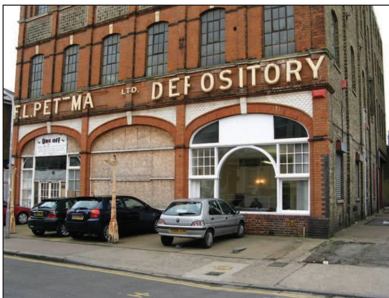
The frontage to the Depository is in need of restoration
